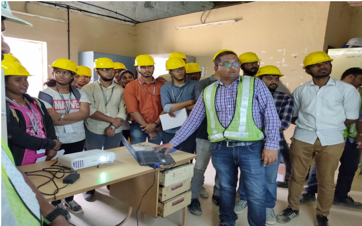
Site Engineer explaining the construction methodology of precast construction technique.
